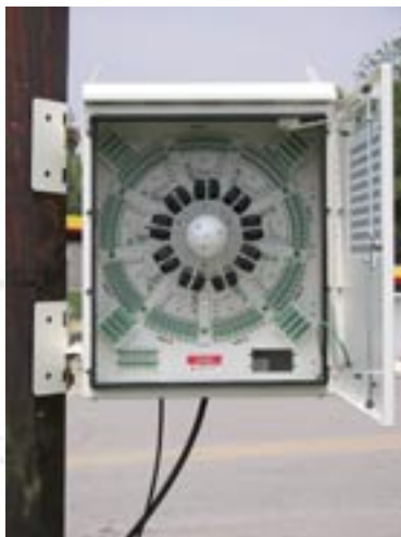
ORBITAL FDC 288 shown in pole mount arrangement
